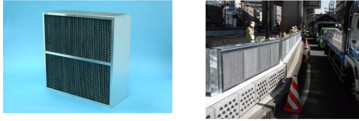
Fig.2. ACF unit for NO x removal and example of the installation at the roadside in Japan
